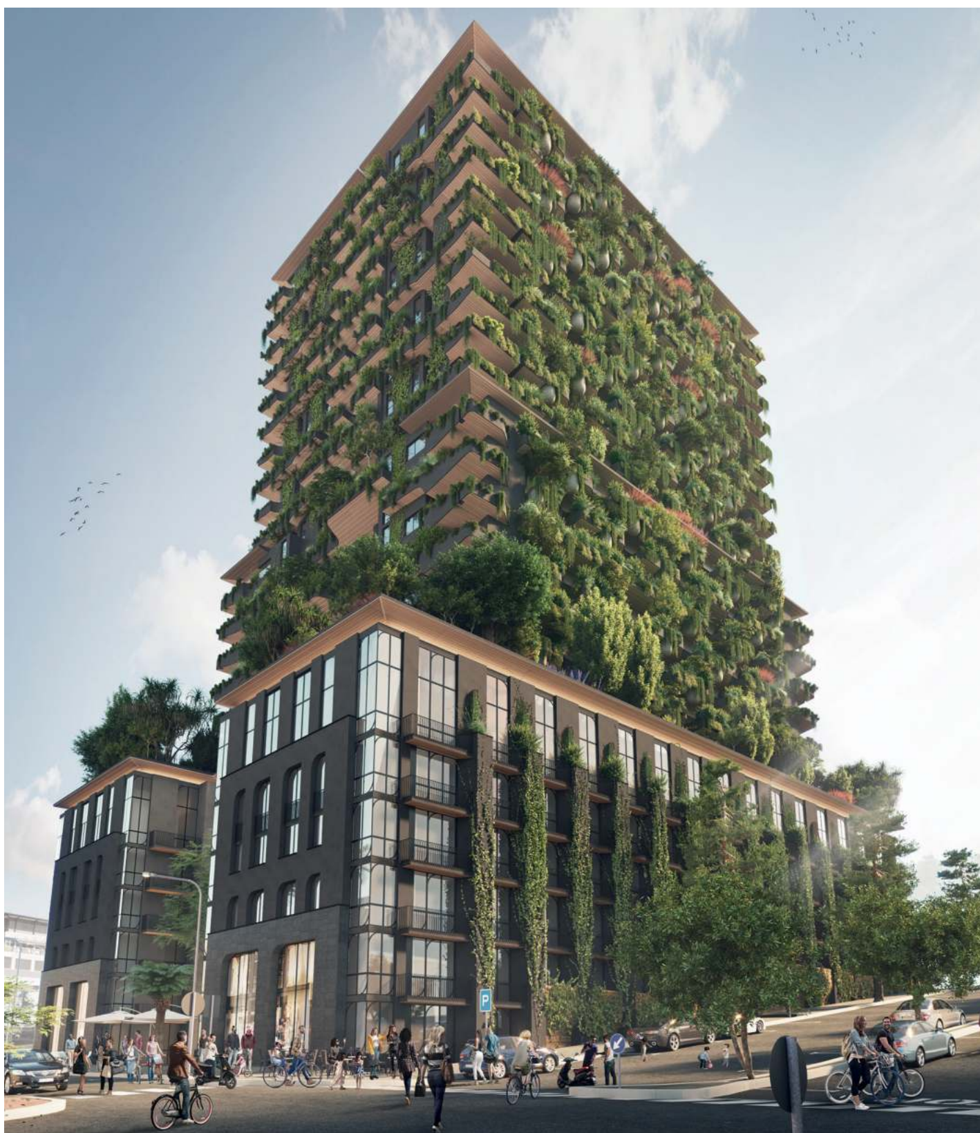
Fynbos, breaking ground in August
